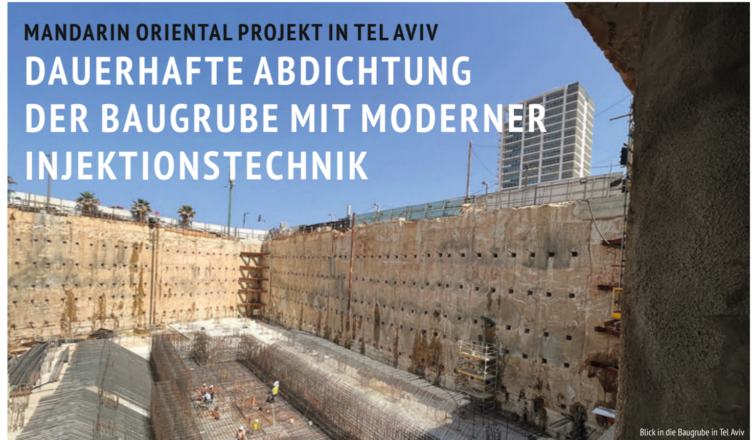
Blick in die Baugrube in Tel Aviv
